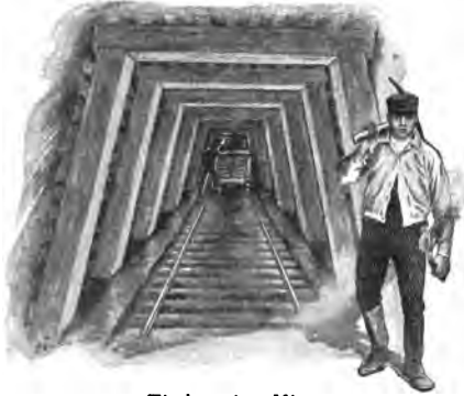
Timbers in a Mine.
